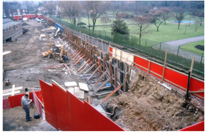
Right: Looking south with Bluebell Steps on the right. The diverted monastic culvert visible bottom centre right shows how the friars' hydraulic engineering survived into the twentieth century.
