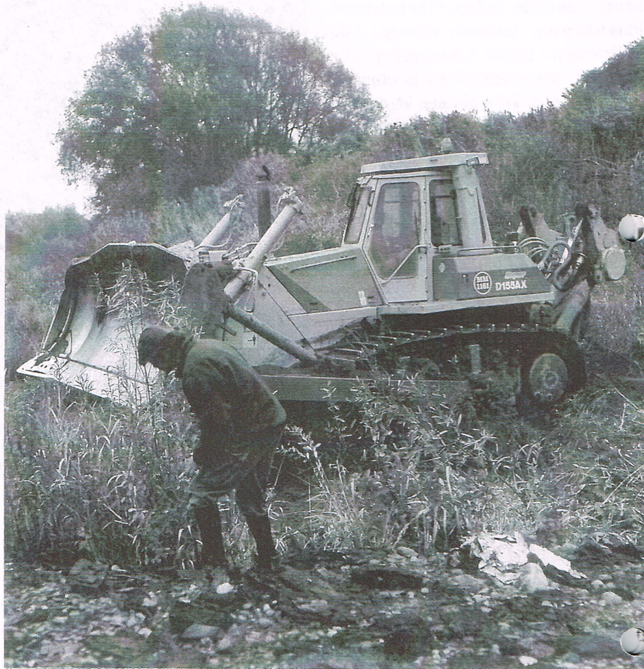
Simon directs the bulldozer with skill and his usual aplomb!
